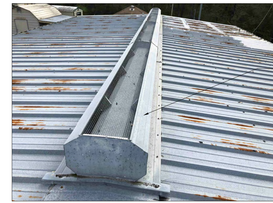
G ROOF VIEW AT RIDGE VENT
