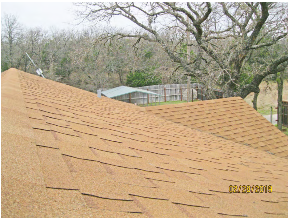
J. View at Vent Thru Roof at Residence
