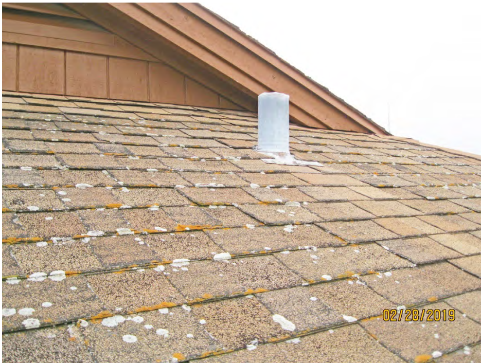
J. View at Vent Thru Roof at Headquarters
