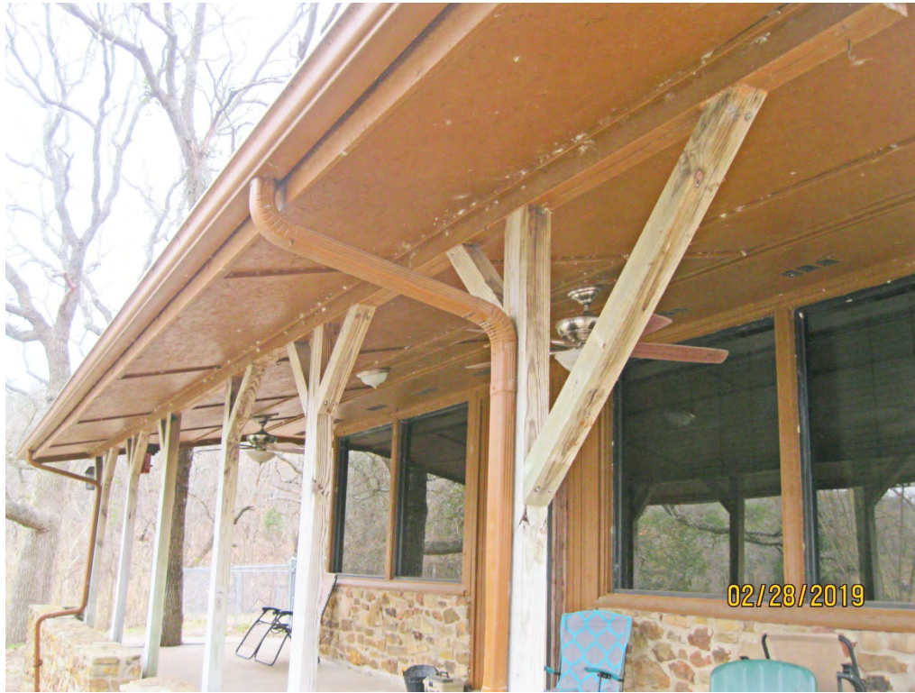
F. View at Gutter and Downspout at Residence
