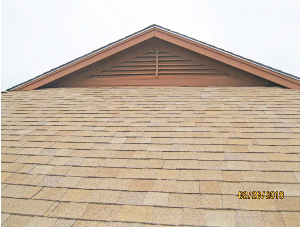
E. View at Headwall Flashing at Training Center
