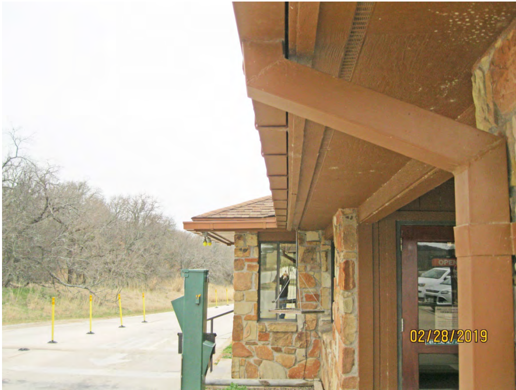
F. View at Downspout and Gutter at Headquarters
