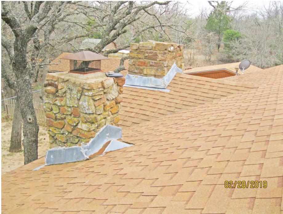
H. View at Chimney at Residence
