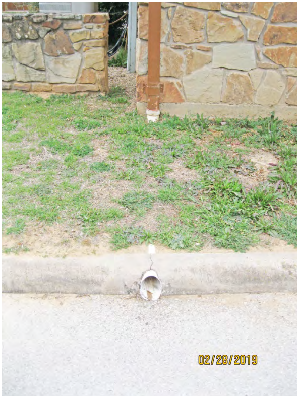
H. View at Existing Drainage at Headquarters
