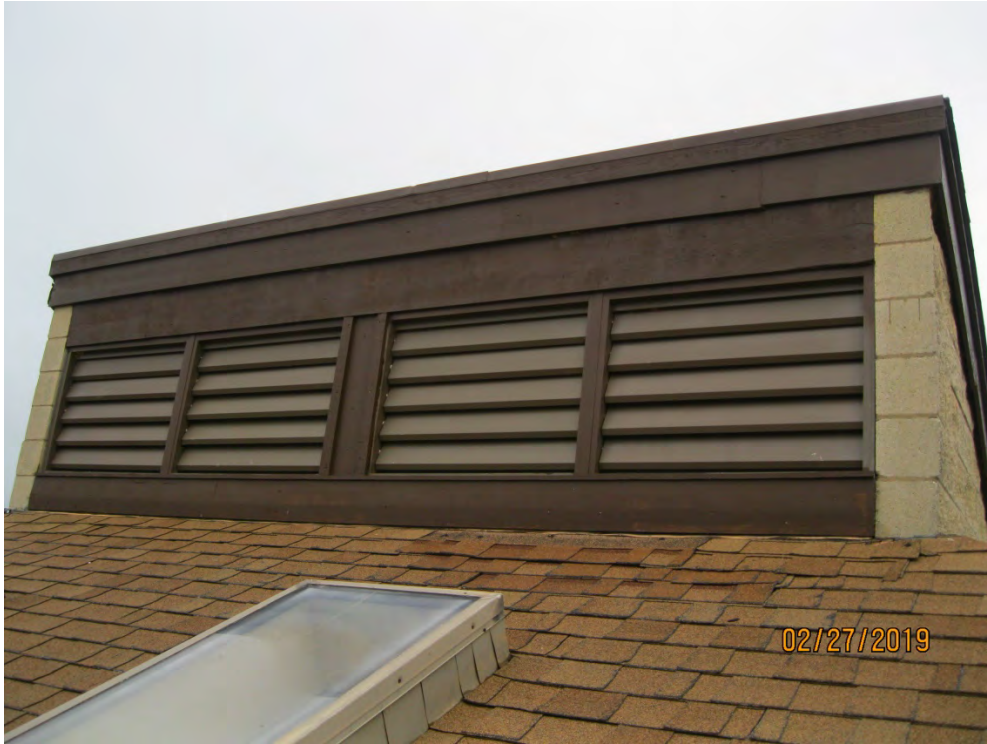
E. View at Headwall Flashing
