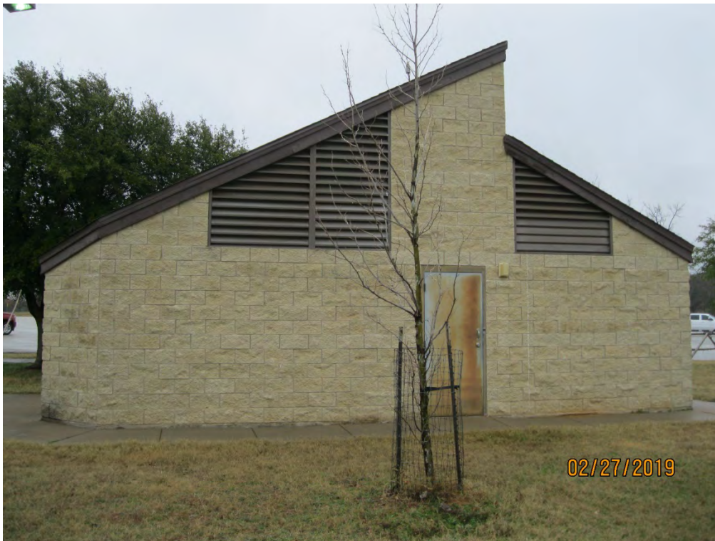
D. East View of IDB Comfort Station
