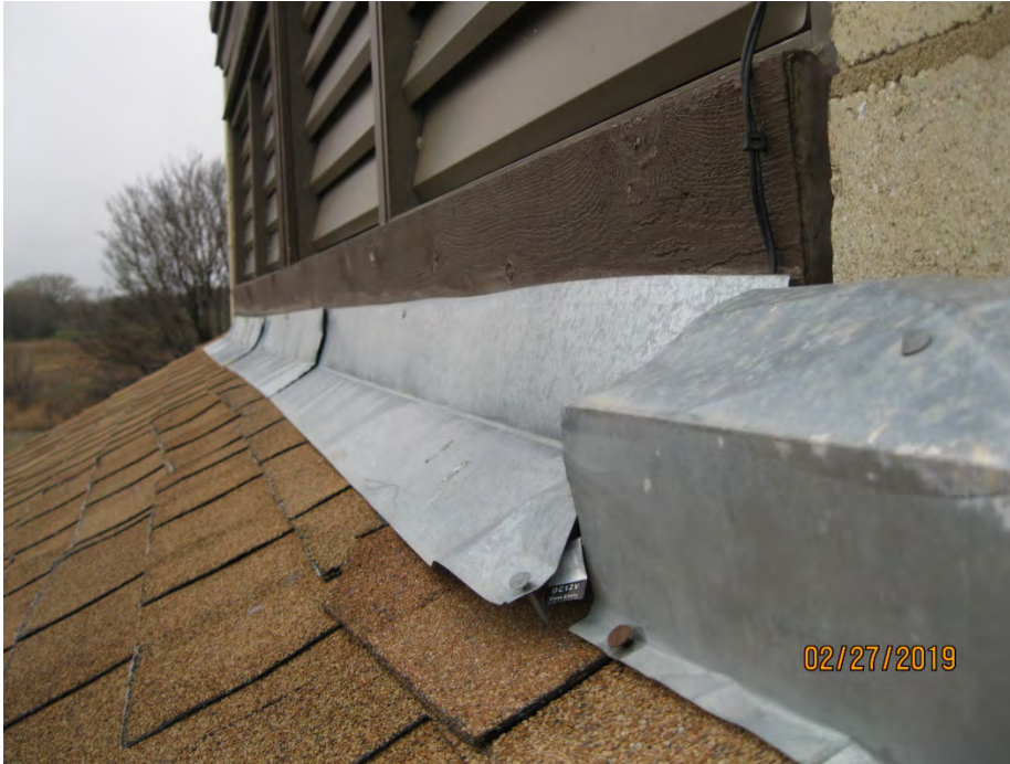
E. View at Headwall Flashing at Greenbelt West Comfort Station
