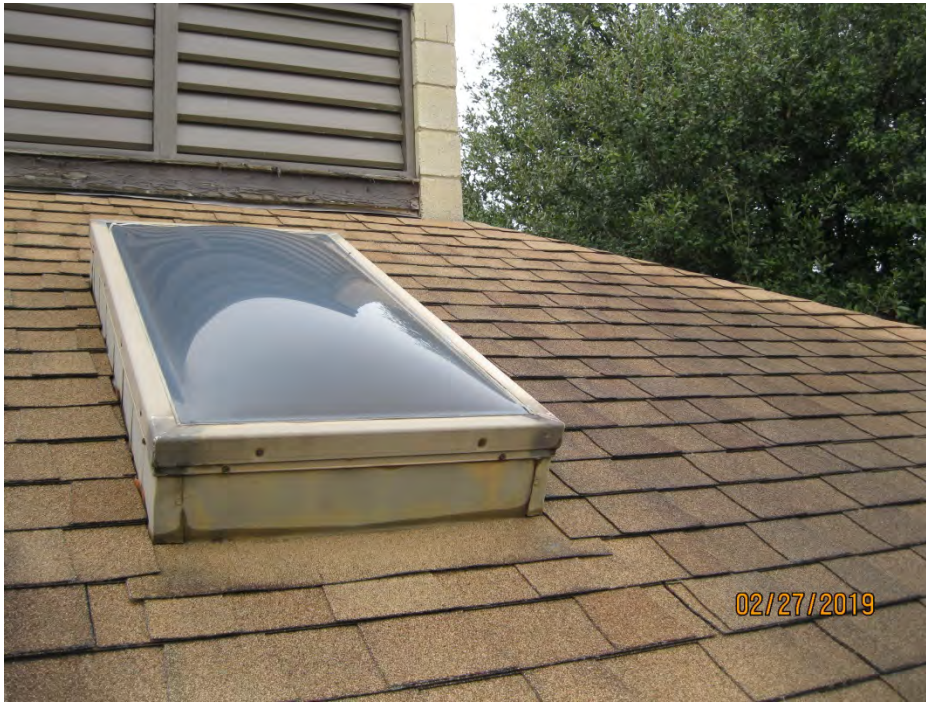
F. View at Skylight at Greenbelt East Comfort Station
