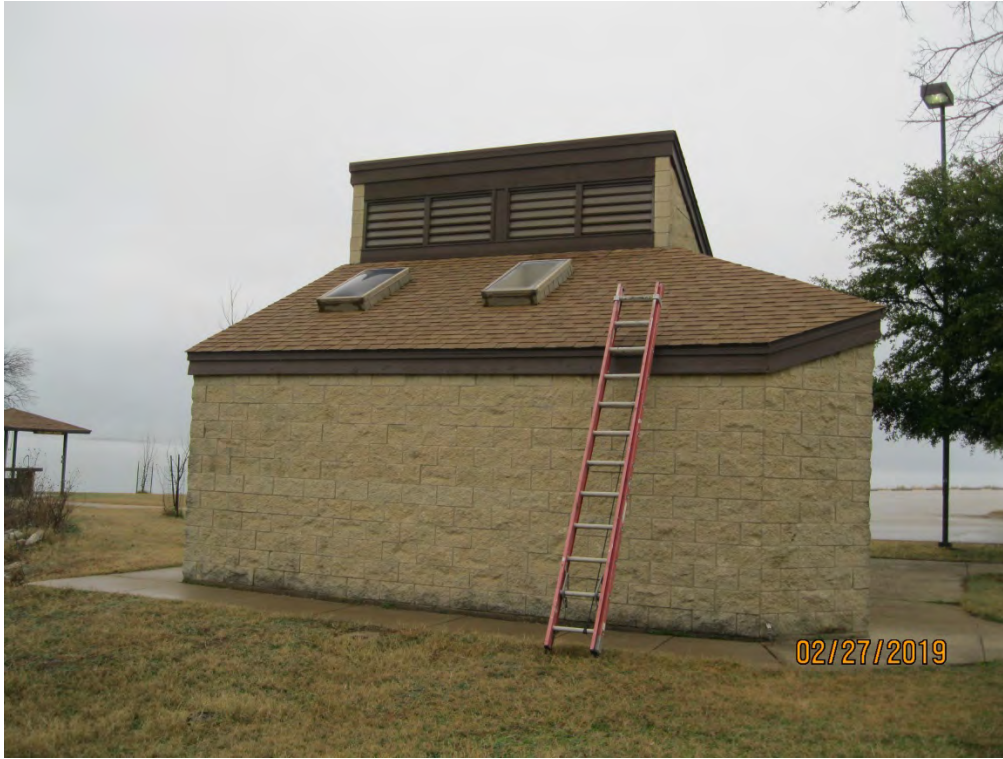
C. North View of IDB Comfort Station
