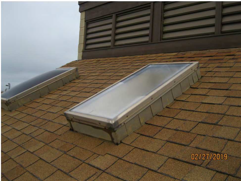
F. View at Skylight
