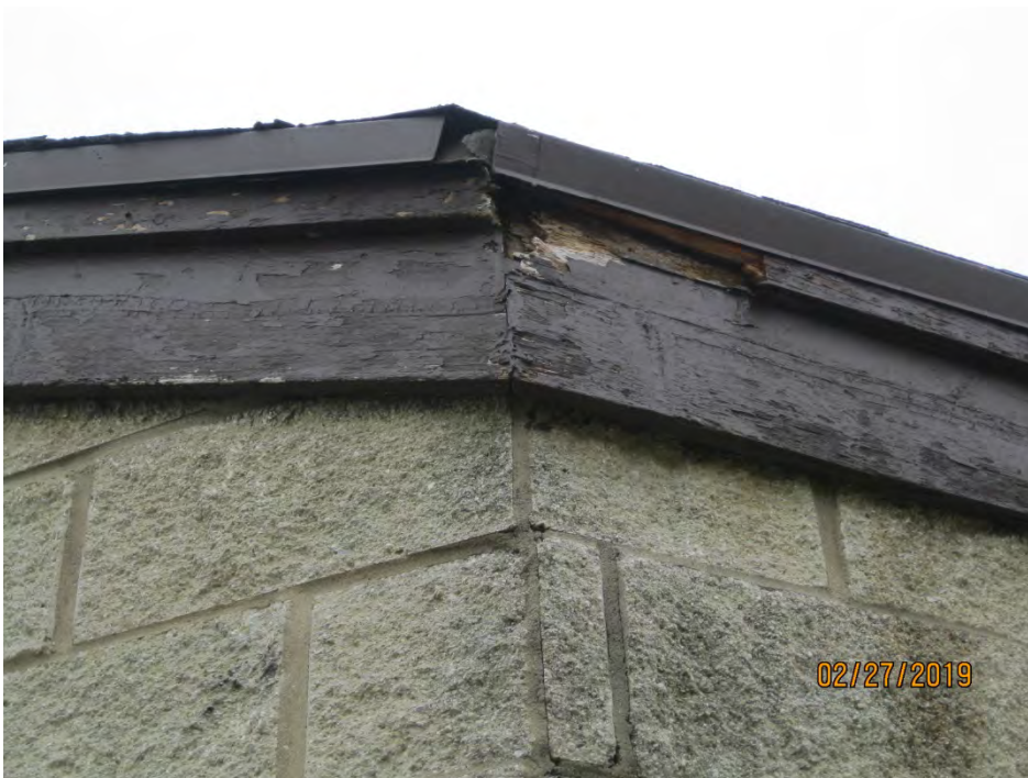
F. View at Rotted Fascia at Greenbelt West Comfort Station
