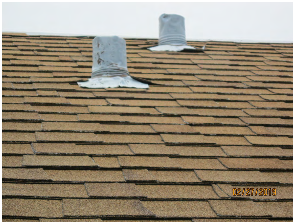
G. View at Penetrations at Greenbelt East Comfort Station
