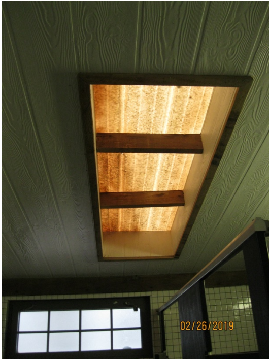
H. View at Skylight at Main Restroom
