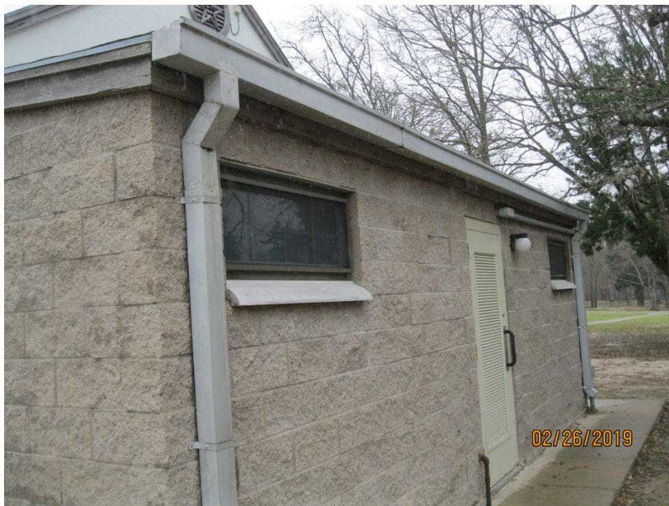
G. View at Gutter and Downspout at Main Restroom
