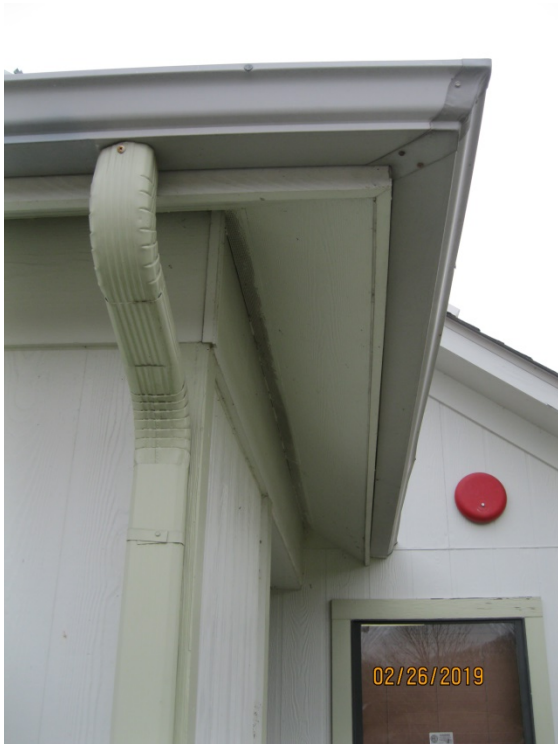
F. View at Typical Gutter and Downspout at Headquarters
