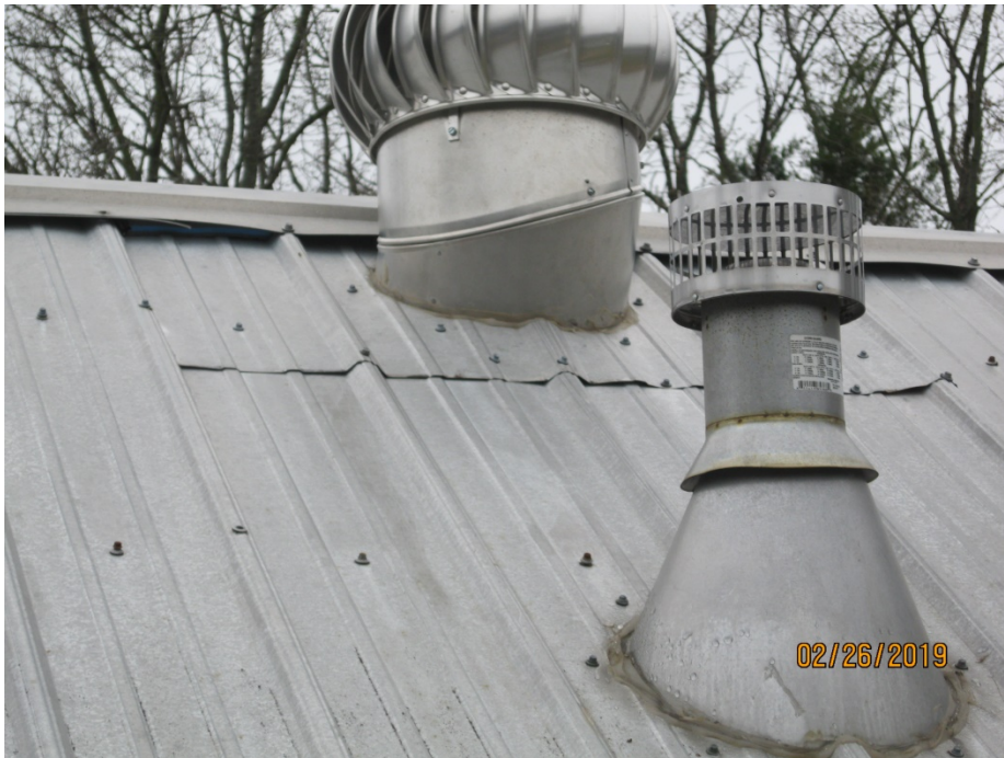
J. View at Penetrations at Main Restroom
