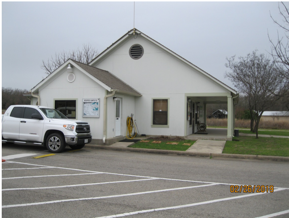
D. East View of Headquarters
