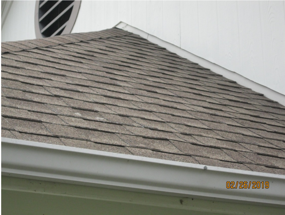
E. View at Sidewall Flashing at Headquarters
