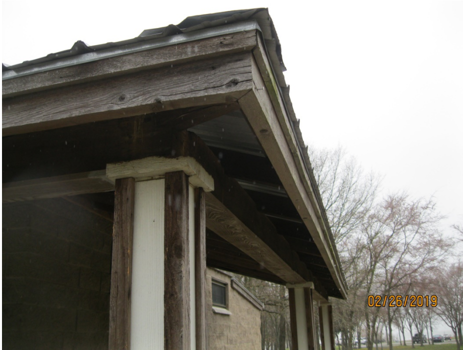
F. View at Typical Fascia at Main Restroom
