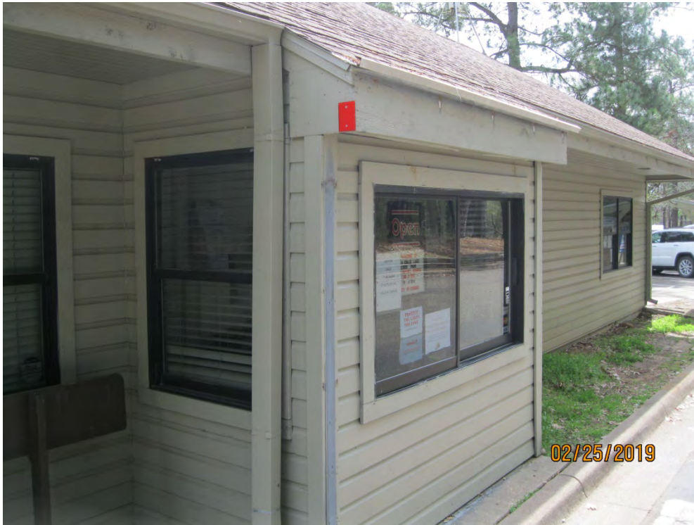
E. View at Drive-up Rake and Gutter at Headquarters
