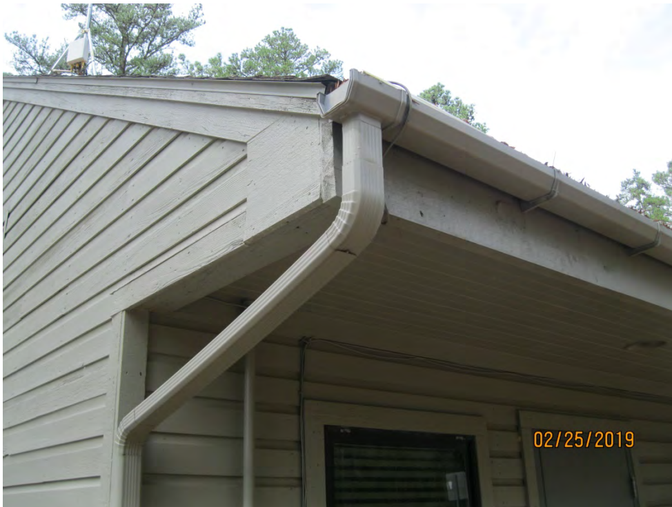
F. View at Typical Downspout and Gutter at Headquarters
