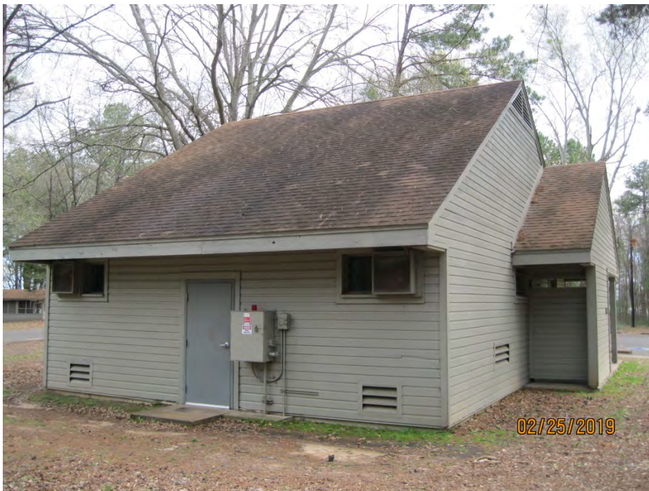
C. Northwest View of Broken Bowl Restroom
