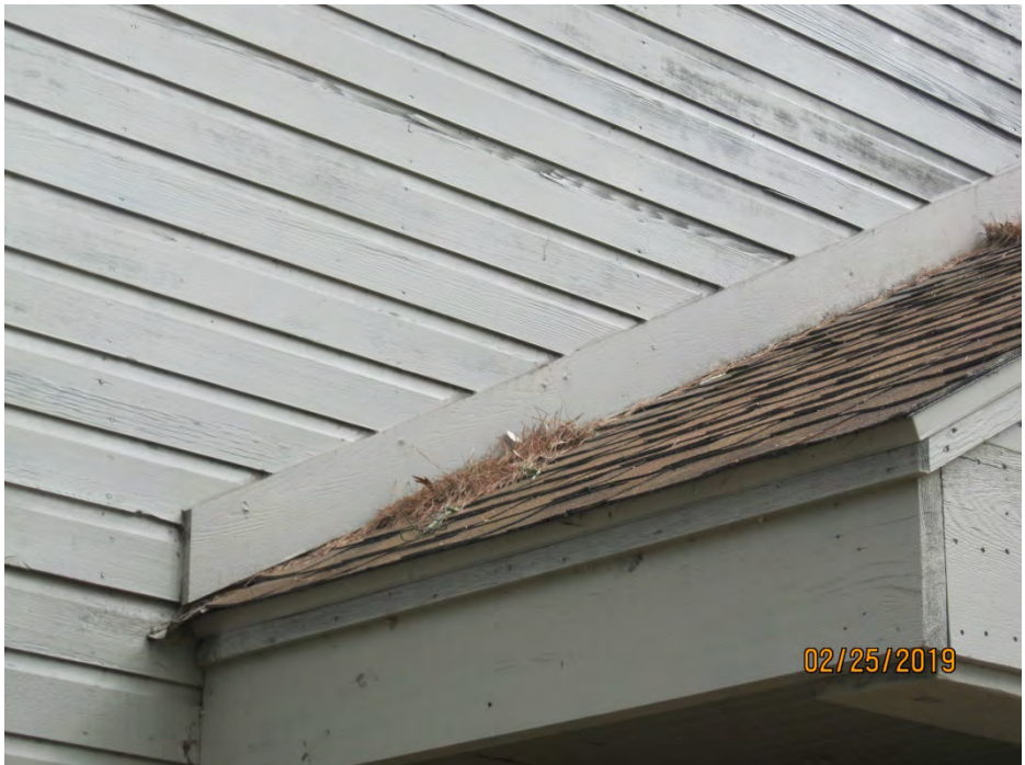
E. View at Sidewall Flashing at Broken Bowl Restroom
