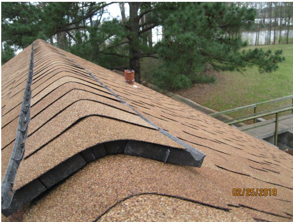
G. View at Ridge Vent at Boat Ramp Comfort Station
