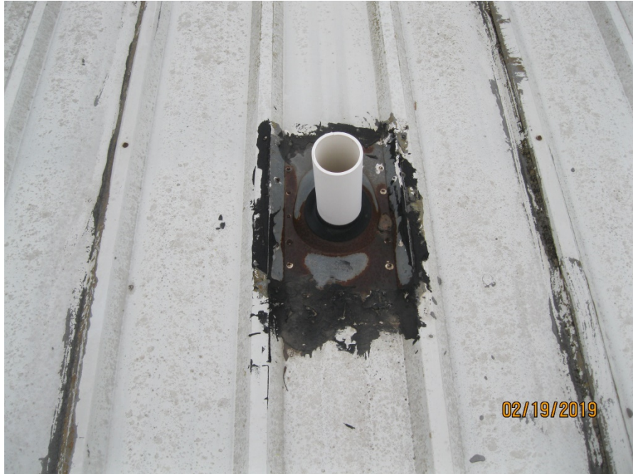
E. Roof View at Existing View through Roof
