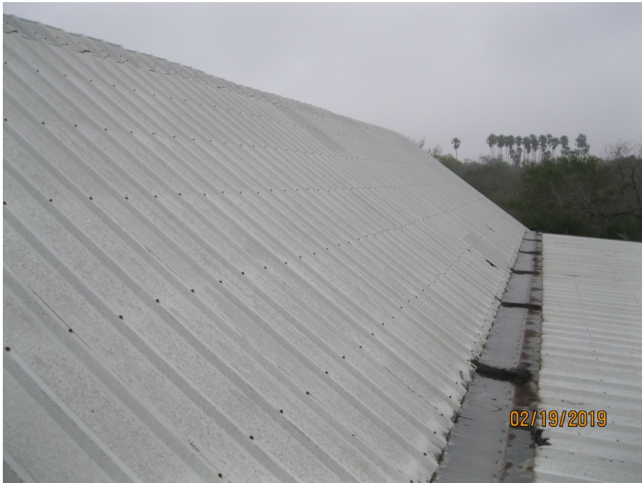
D. Roof View at Slope Transition Flashing
