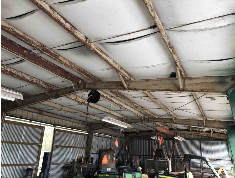
E. View of Purlins
