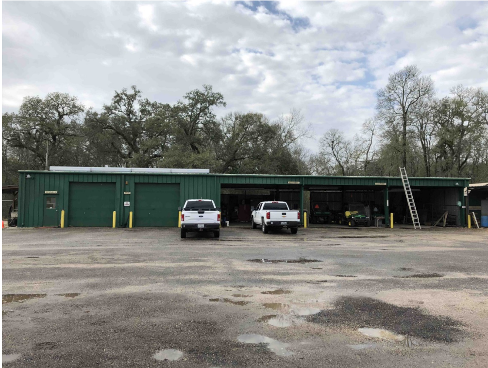
C. North View of Maintenance Shop
