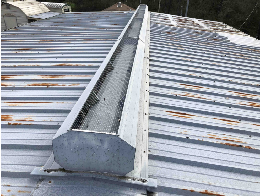
H. Roof View at Vent Thru Roof
