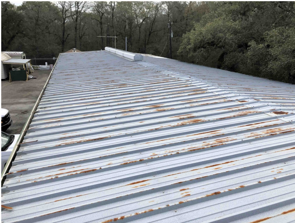
F. Roof View Looking East
