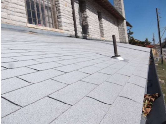
(HA-25) No Asbestos Detected
