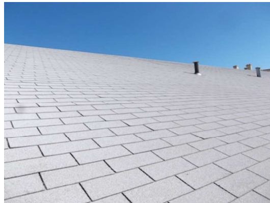
(HA-04) No Asbestos Detected
