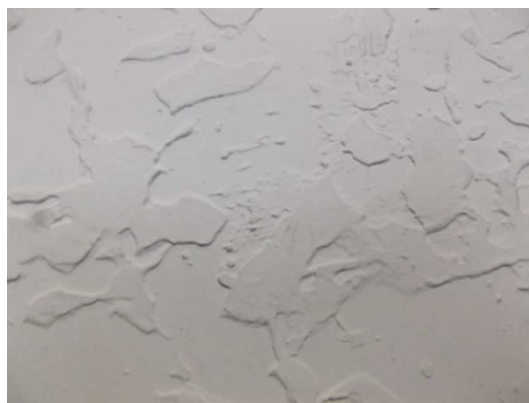
(HA-22) No Asbestos Detected
