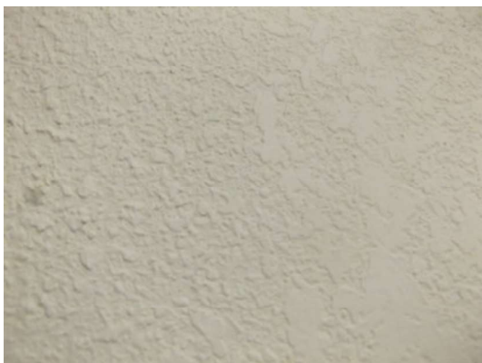
(HA-23) No Asbestos Detected
