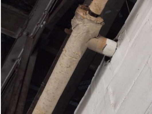
(HA-07) No Asbestos Detected
