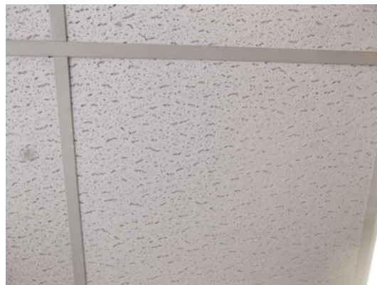
(HA-06) No Asbestos Detected
