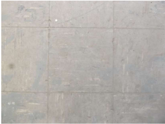
(HA-01) Asbestos Detected
