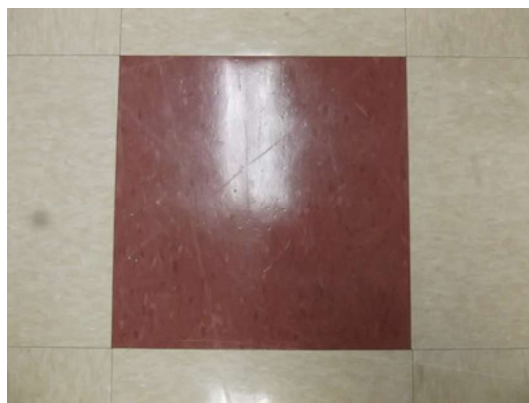
(HA-10) No Asbestos Detected
