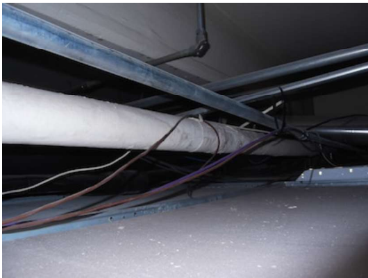
(HA-27) Asbestos Detected
