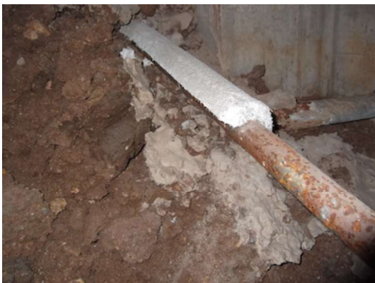
(HA-05) Asbestos Detected
