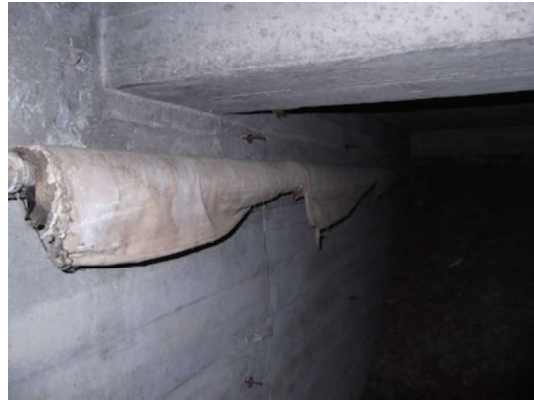
(HA-04) Asbestos Detected
