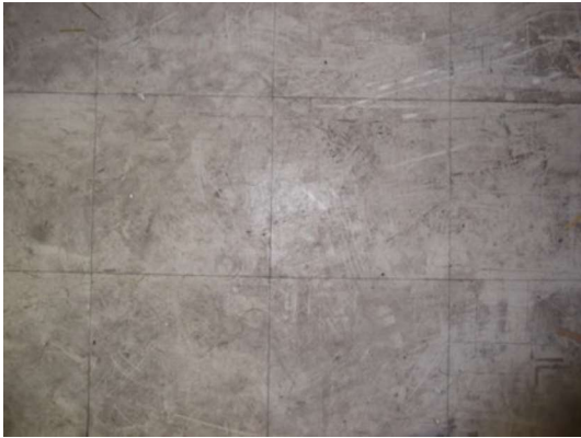
(HA-01) Asbestos Detected
