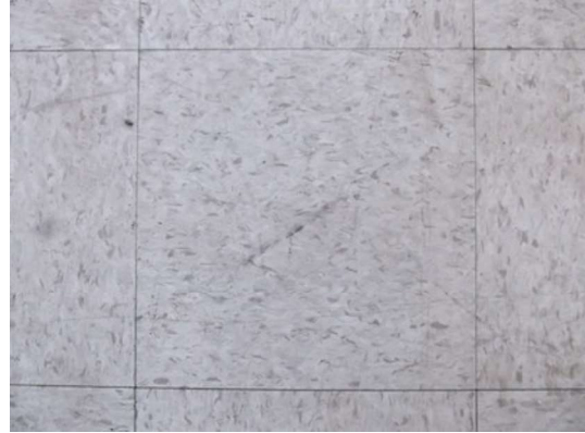
(HA-02) Asbestos Detected
