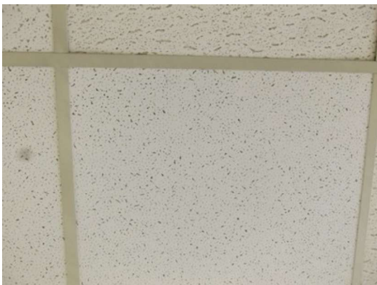
(HA-05) No Asbestos Detected
