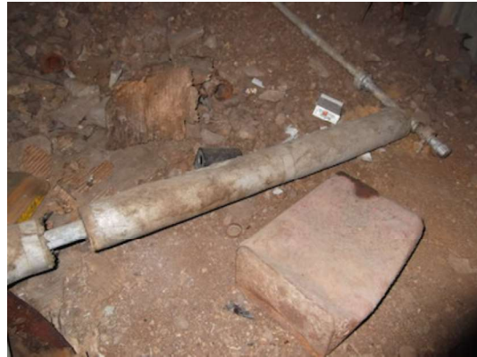
(HA-04) Asbestos Detected
