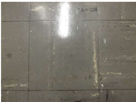
(HA-11) Asbestos Detected
