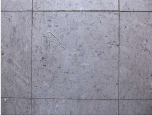
(HA-01) Asbestos Detected
