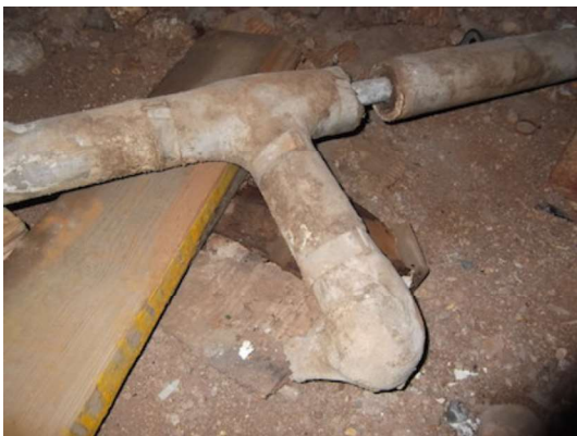
(HA-05) Asbestos Detected
