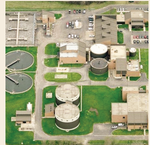
Woodridge Greene Valley Treatment Plant
