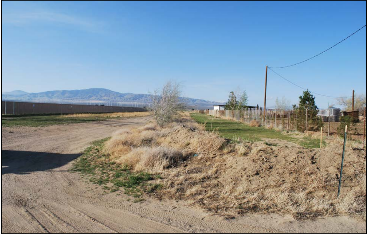
Photo 15: Section 4B, view north along 150 th Street W from W Avenue A
