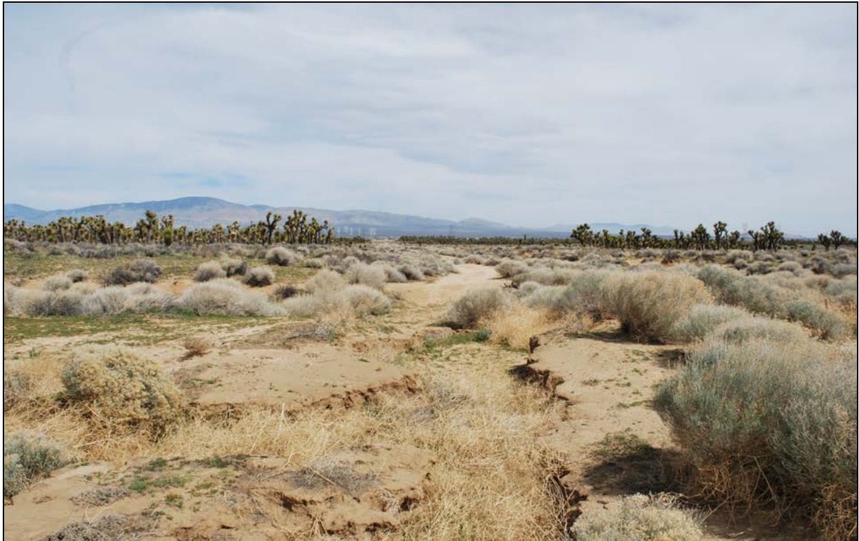
Photo 20: Section 7, view north along 155 th Street W from W Avenue C
