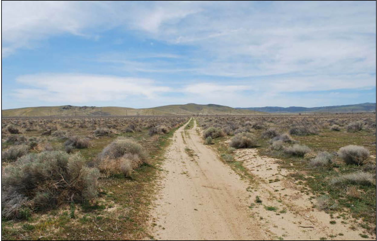
Photo 21: Section 7, view south along 155 th Street W from W Avenue C
