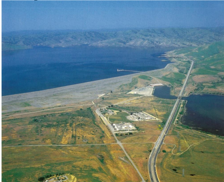
Figure 7: Aerial View of San Luis Reservoir
