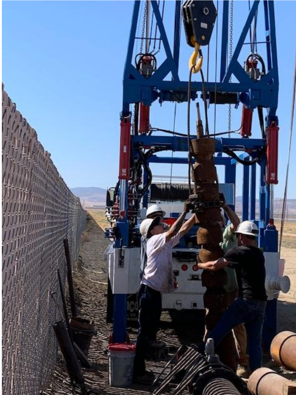
Figure 8. Pump Bowls and Impellers
