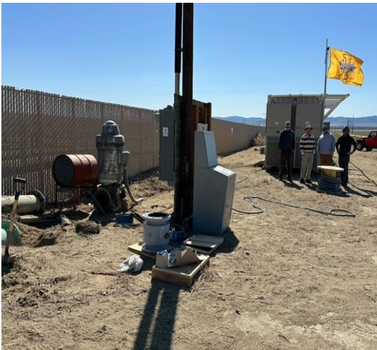
APH site with Container
