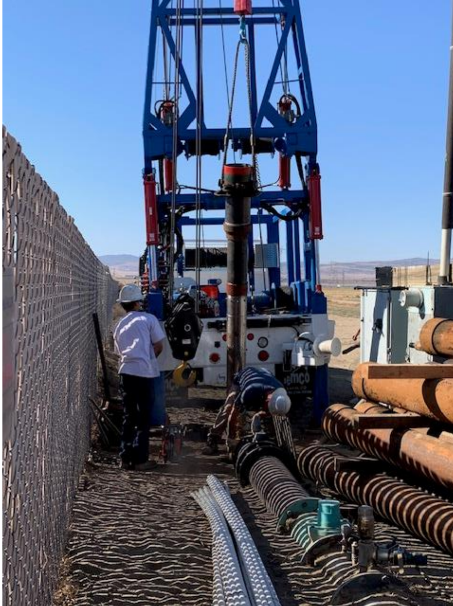
Figure 11. APH Valve Installed at Bottom of Pipe Column
