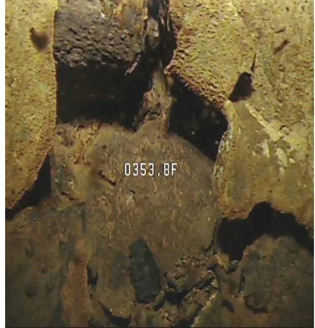
Figure 6. Patch and Obtrusions at 353 Ft.
