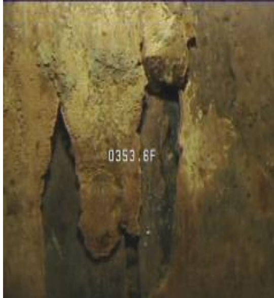
Figure 6. Patch and Obtrusions at 353 Ft.
