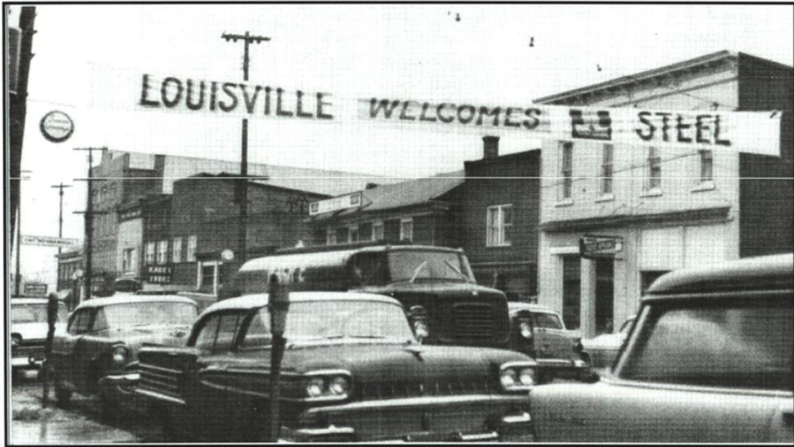
FIGURE 12: E. Main, looking northwest - 213-217 E. Main in foreground, 1959, from Stainless & Strip
