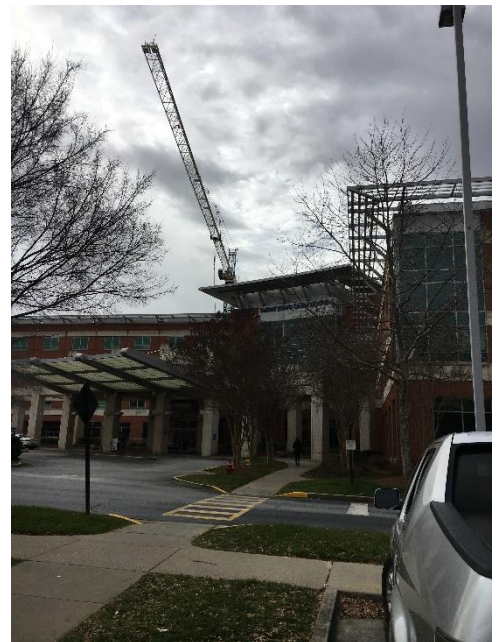
Cranes Setting Beams January 10, 2020
