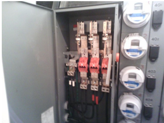
Picture No.9-b: 4 th Floor Disconnect at the Electrical Room
