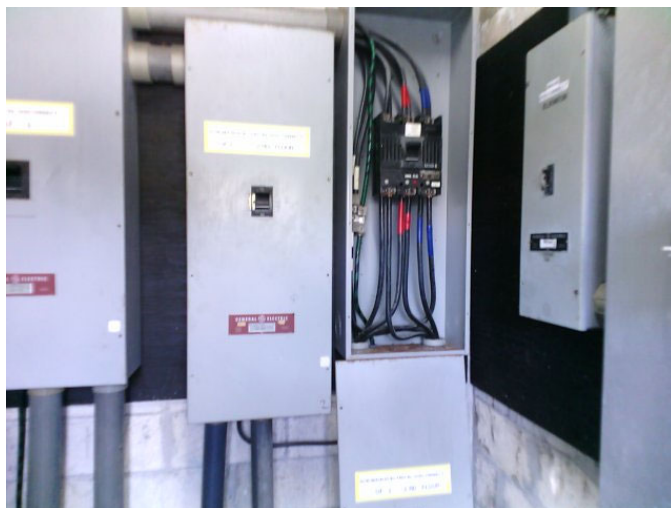
Picture No.6-b: Disconnect 2 of 2 (3 rd Floor) at the Electrical Room 1 st Floor
