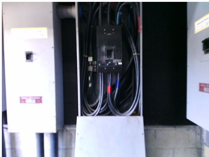
Picture No.3-b: Main Disconnect 1 (4 th & 5 th Floor) at the Electrical Room 1 st Floor
