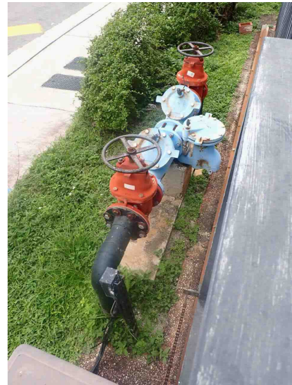
fire sprinkler backflows
