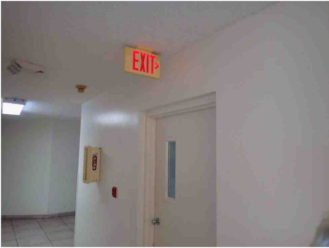
fire alarm pull station, lit emergency exit sign, extinguisher
