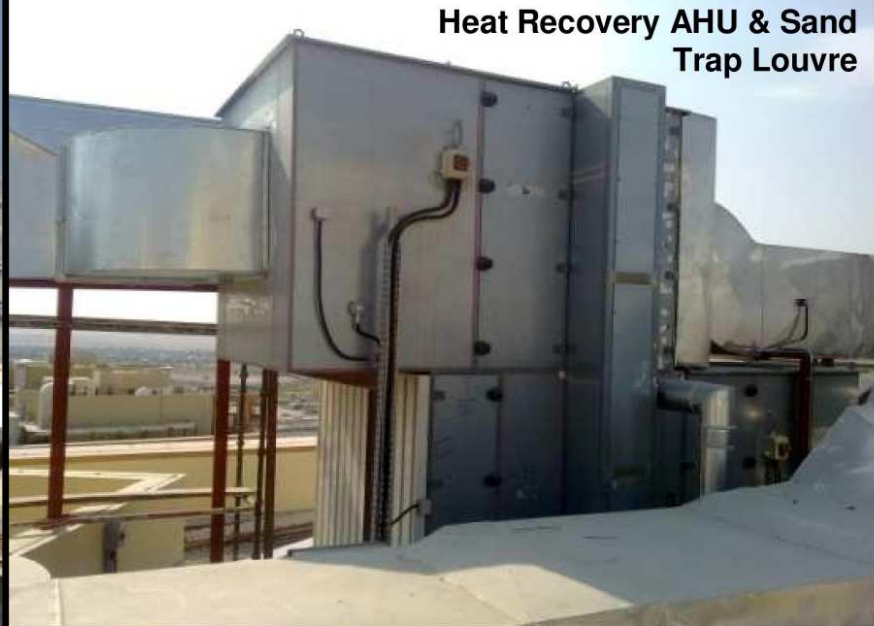
SA/RA GI Ducting with Fibre glass Insulation, Canvas cloth, Foster & Aluminum Cladding
