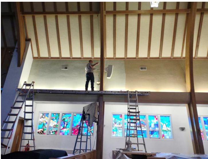
Troy Bachtle - Building manager, painting the second tier of the Sanctuary walls
