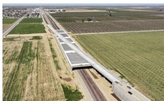
Finished viaduct in 2024.
