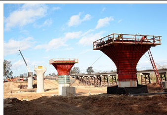
The Fresno River Viaduct, part of the IOS, under construction, 2016.
