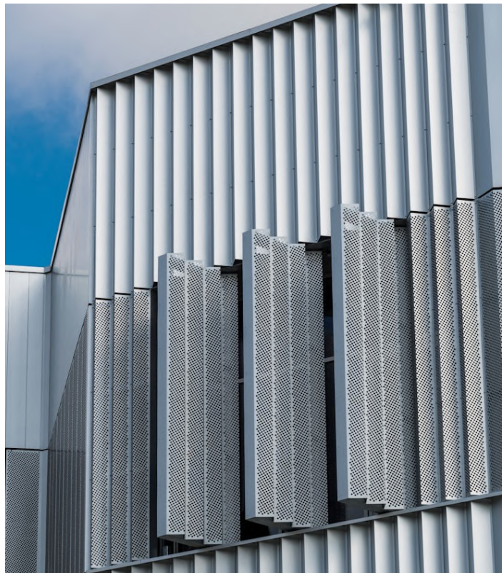
Deca Packaging - Herentals Architect: 2DVW architecten bvba
