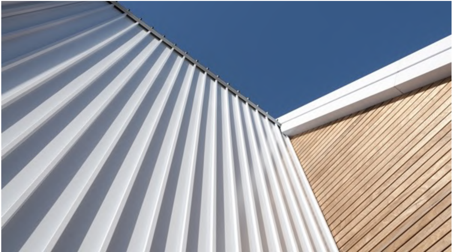
Gymnasium Kernhem - liner roof - Ede Architect: Strategie Architecten
