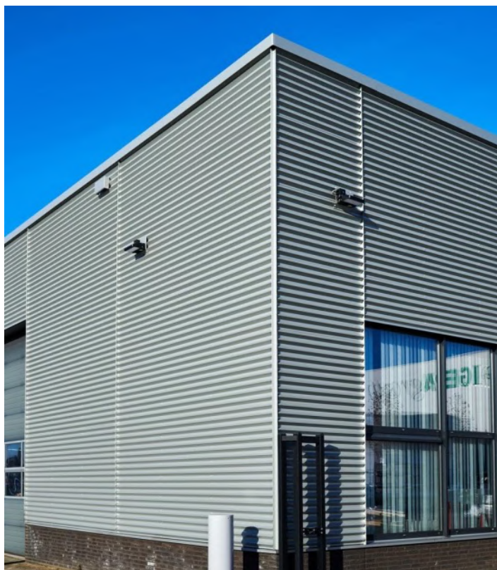
ISIS Custom-made - Renovation Tiel Hairexcel 6906 (9006)
