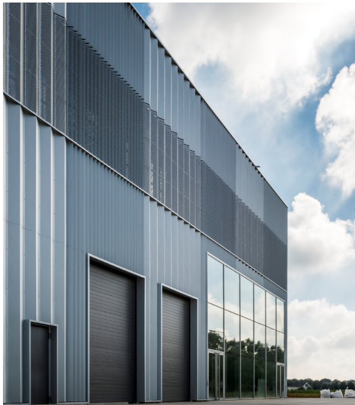
Deca Packaging - Herentals Architect: 2DVW architecten bvba
