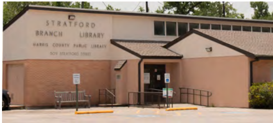
Figure 1.2.3 Surrounding Libraries (Photos: Harris County Public Library)
