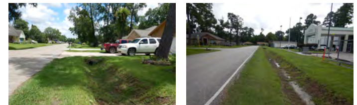
Figure 3.24 Existing Condition - Ditches
