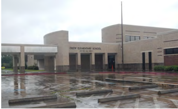
Photo 6: Drew Elementary School
