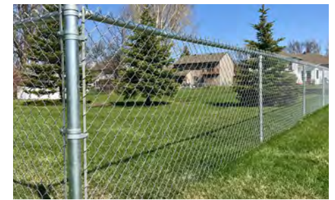
Removing chainlink or unsteady fencing and applying durable materials
