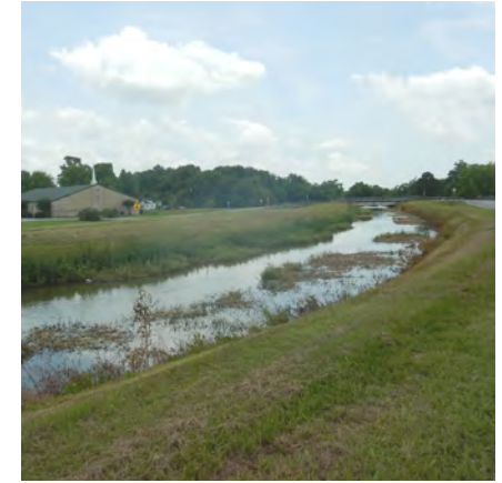
Figure 3.79 Existing Site Context
