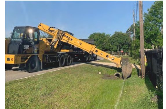
Figure 2.1.14 Ditch Cleaning/Vactoring
