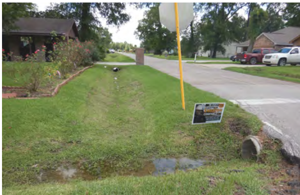
Figure 1.3.18 Existing Drainage Conditions
