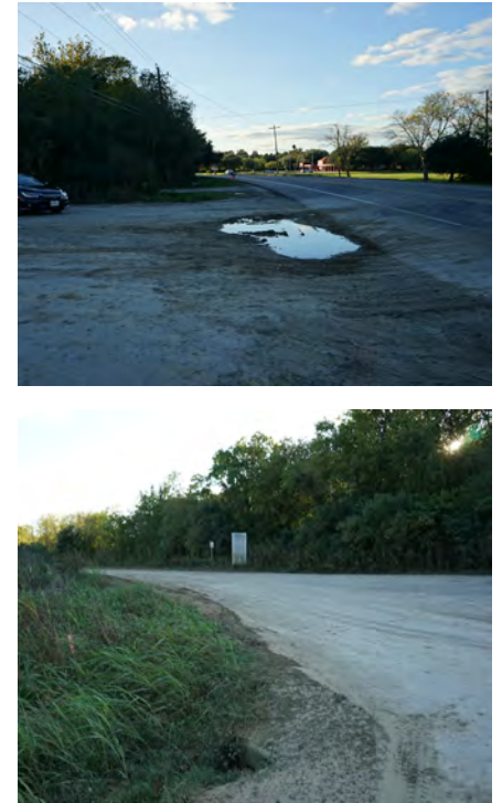
Figure 3.62 Existing Conditions - Eagleton Lane and FM 1942 Intersection
