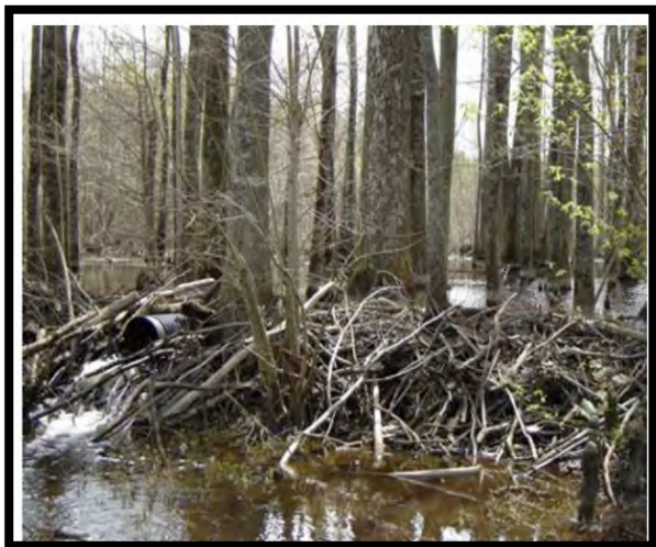
Figure 35: Flexible pond levelers with cylindrical wire cages on the upstream pipe end. Clockwise from upper left (a) and (b) are examples during the construction phase, while (c) is an example just after completion but before dam repair. (b) is a downstream view of a pond leveler after beaver have repaired the dam. Photographs from Boyle (2006).
