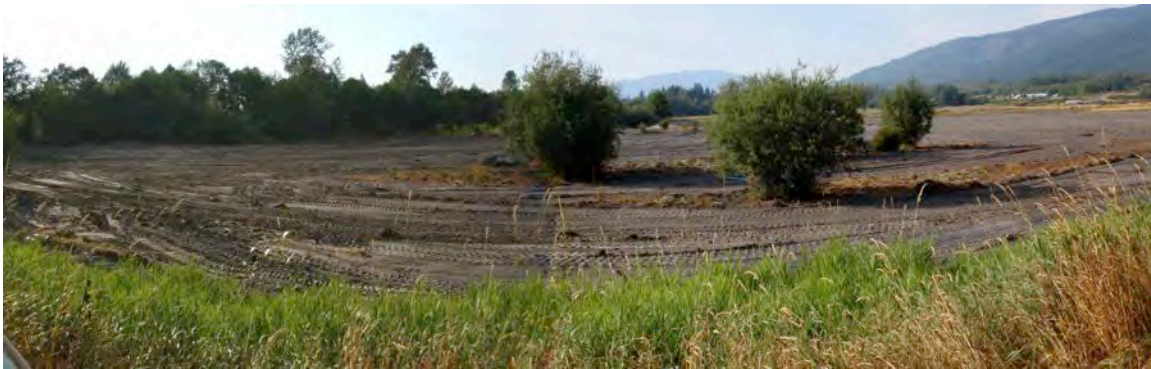
Figure 80: Photo of the restoration site during construction after removal of invasive reed canarygrass
