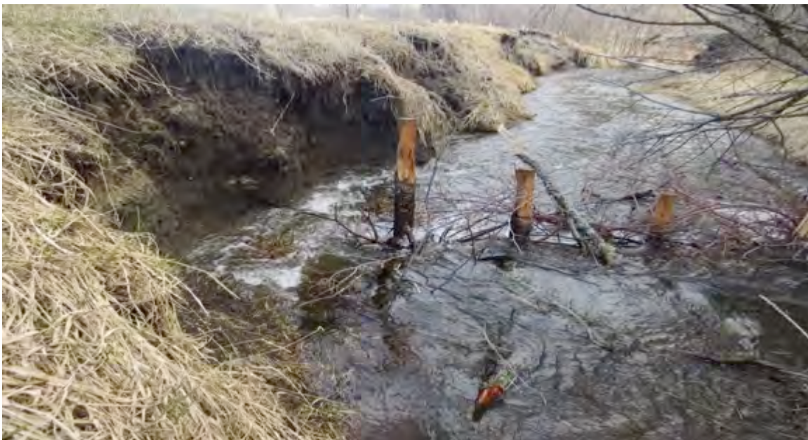
Figure 78: Breach of BDA 1 showing water flowing around the structure, eroding the left bank. This BDA is still functioning as grade control through water impoundment upstream as well as facilitating the widening of the incision trench. Notice the development of an inset flood plain directly downstream along the right bank
