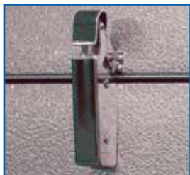
Spring actuated door closer
