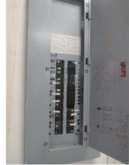
1st Flr Electric Panel Box
