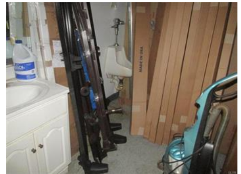
1st Flr Rest Room
