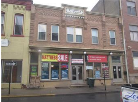
Front of building
