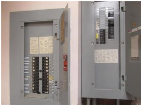
2nd Flr Electric Panel Boxes
