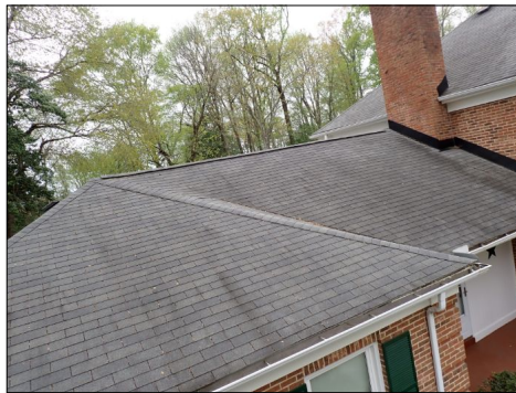
Asphalt Shingles
