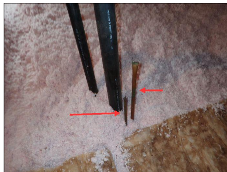
Plumbing Rough In
