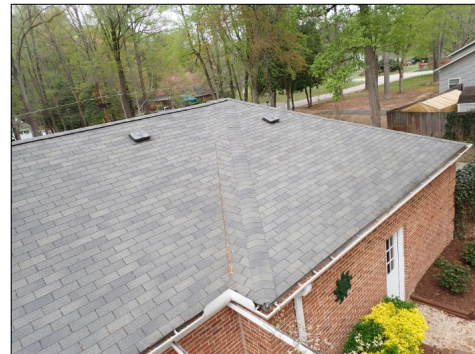
Asphalt Shingles
