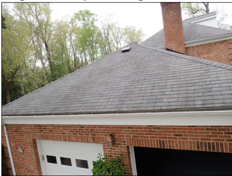
Asphalt Shingles
