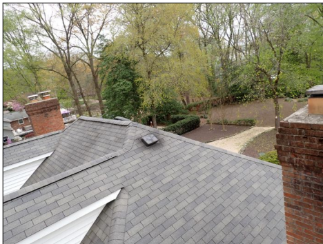
Asphalt Shingles
