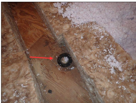
Toilet Rough In
