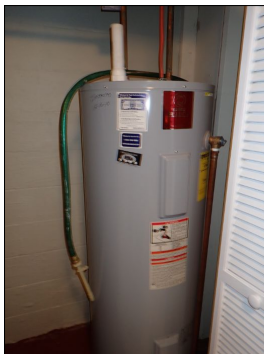
Electric Water Heater
