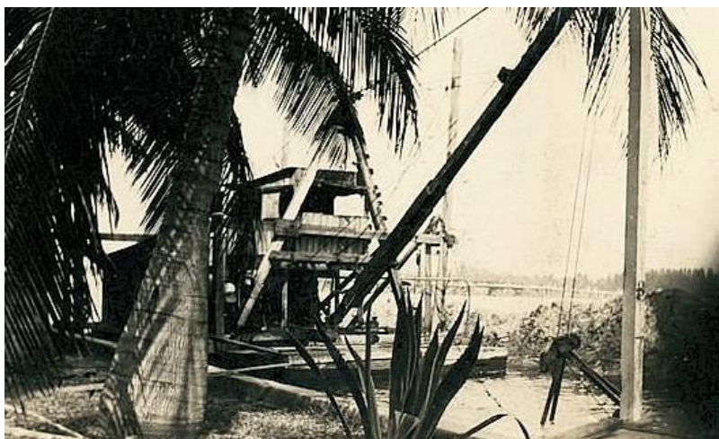
Figure 9 Steam-powered dredgers like this connected the Loxahatchee River to Lake Worth, as well as the new and deeper 1920 Palm Beach Inlet. Courtesy Historical Society of Palm Beach County
