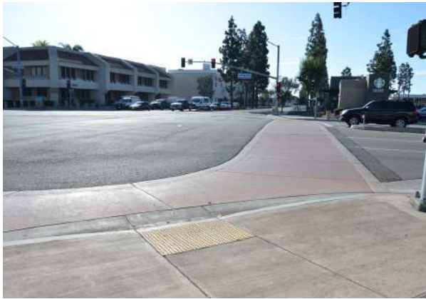
Colored concrete pavement material used at major intersection pedestrian crossings for Euclid Street and Garden Grove Boulevard can lack visibility and contrast.
