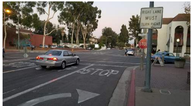
Multiple approaches at existing all-way stop (Acacia Parkway & Main Street) intersections can limit traffic flow and impact safety of other roadway users.
