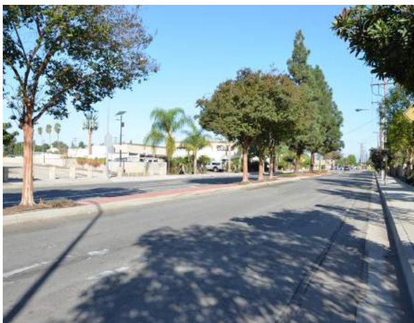
Wide travel lanes present opportunities for traffic calming and accommodation of bikeway facilities.
