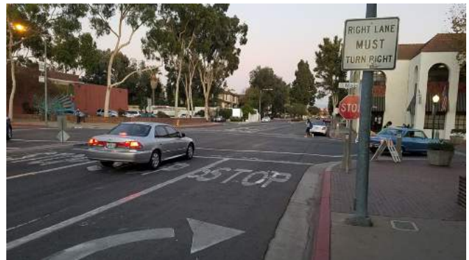
Multiple approaches at existing all-way stop (Acacia Parkway & Main Street) intersections can limit traffic flow and impact safety of other roadway users.
