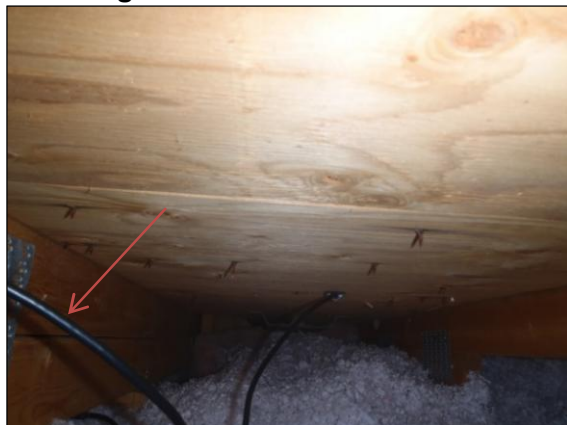
Figure B.21: Unit 3 east truss
