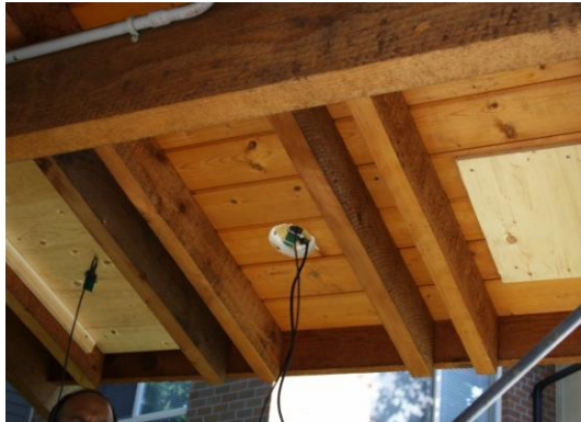
Photo 14: Control Assembly Sensors
