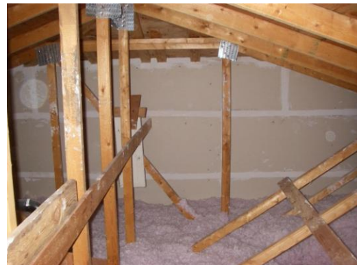
Photo 9: Drywall Fire Separation
