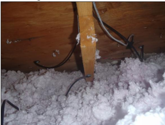
Figure B.5: Unit 1 east truss
