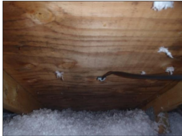
Figure B.26: Unit 4 north non-baffle
