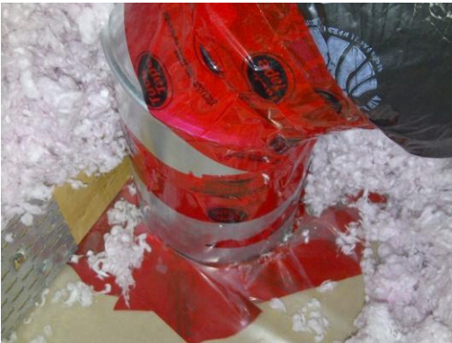
Photo 6: Air Barrier Sealing of Dryer Duct Penetration at Ceiling
