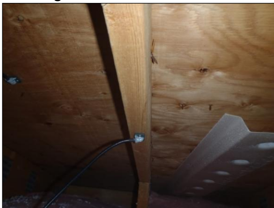
Figure B.29: Unit 4 south truss
