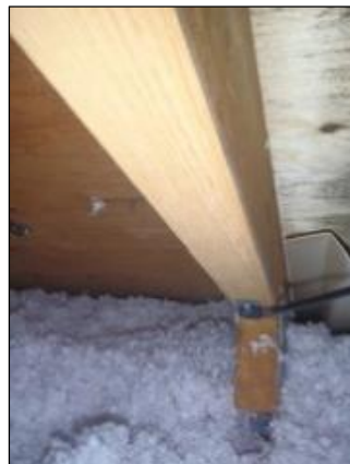
Figure B.22: Unit 3 west truss
