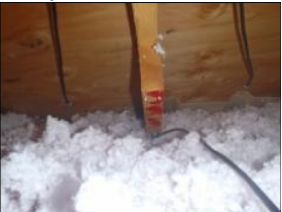
Figure B.6: Unit 1 west truss
