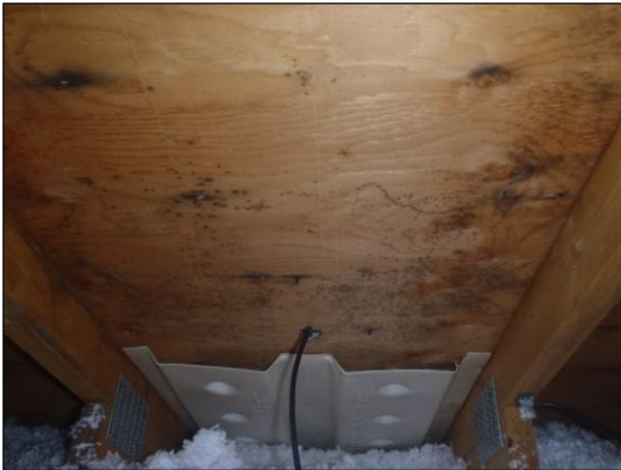
Figure B.9: Unit 2 east baffle
