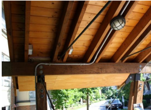
Photo 15: Control Assembly Data Outdoor Air Measurements
