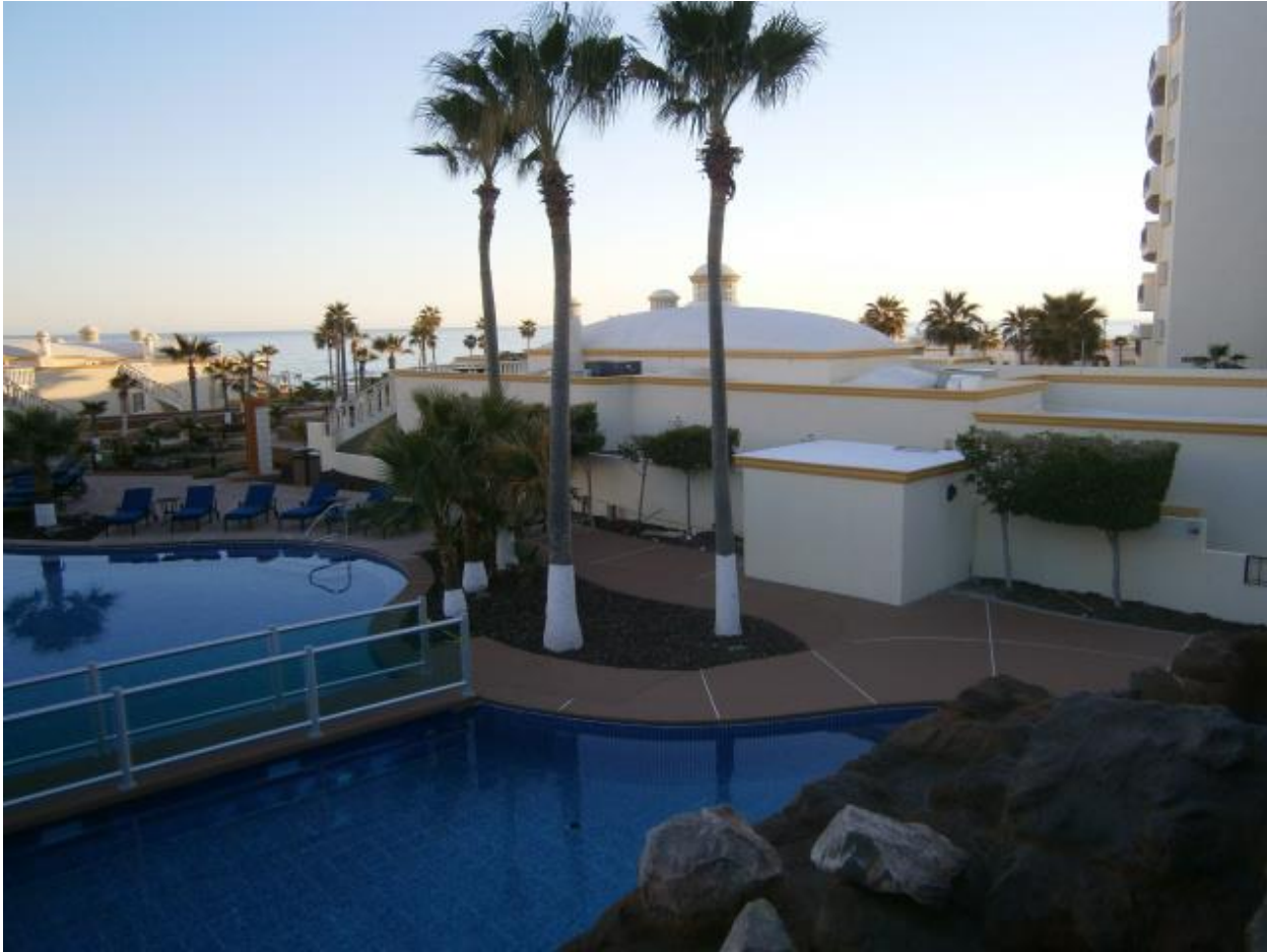
The Baja Building rails have been completed, and the yellow trim removed.
