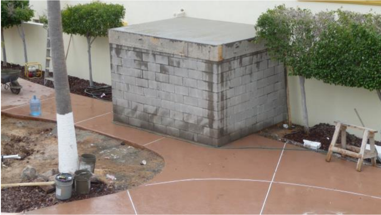
The new pump room to house the new heater and pumps. Power is being run and matching stucco is next..
