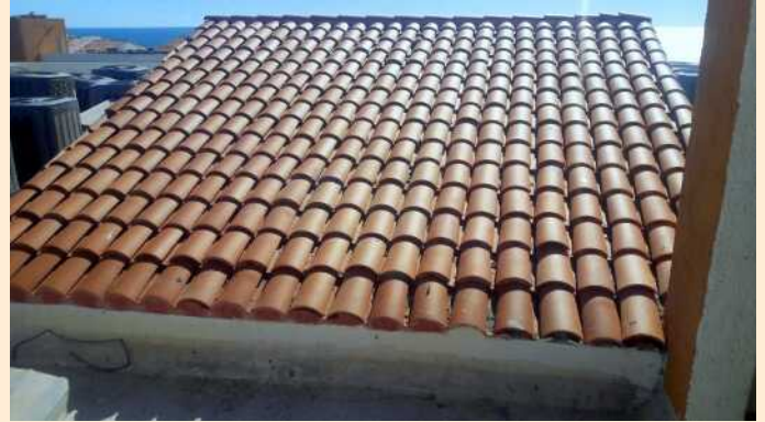
After Tiles Replaced
