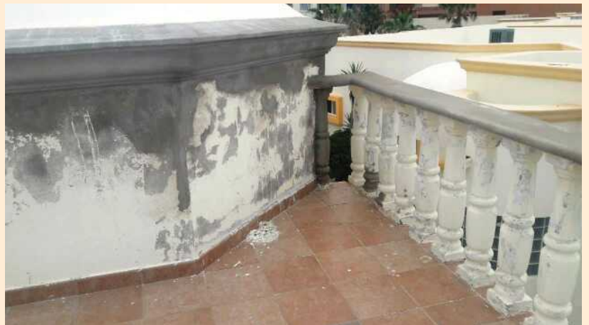
Maintenance and Paint Touch Up on Villas
