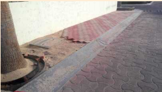
New pavers at Delphin & Baja
