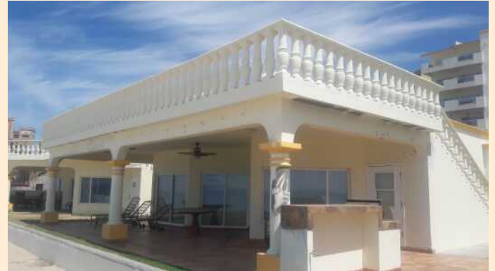
Repair of Pillars and Paint Touch Ups
