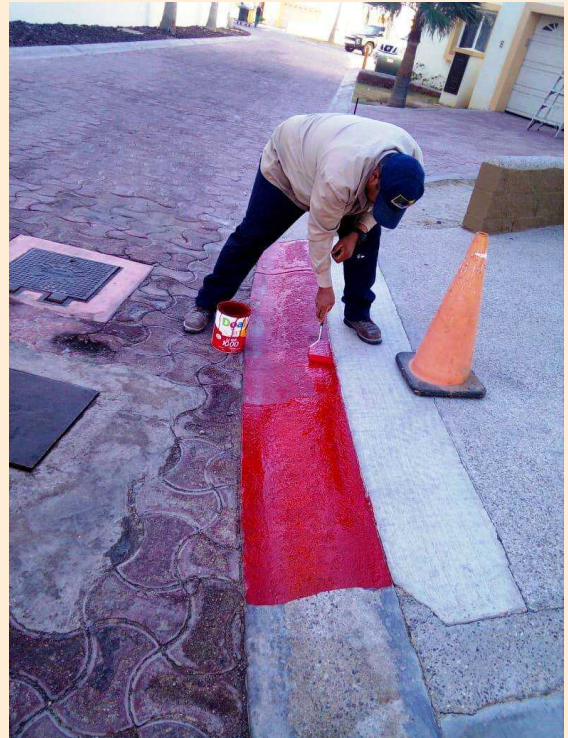
Curb repair & paint Touch Up On curbs
