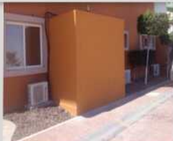
Cable-TV Internet Control Room for high speed internet and TV service
