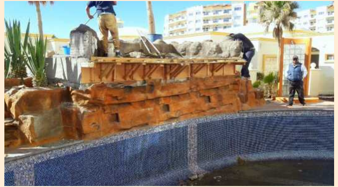
Baja Pump Room Ceiling Repair
