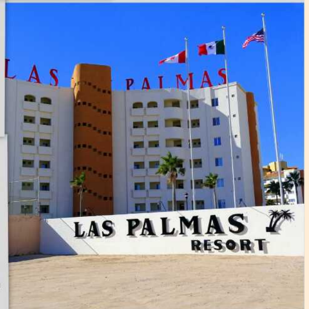
New Entrance Sign with Tri Country Flag Poles
