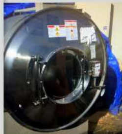
Commercial Laundry Equipment added to new laundry room
