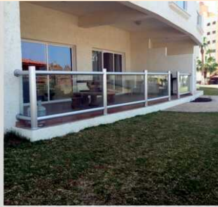
Alumimum and Glass Raiings replaced rusting wrought iron
