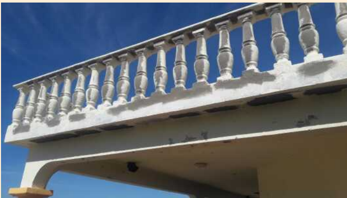
Repair of Pillars of the Villas
