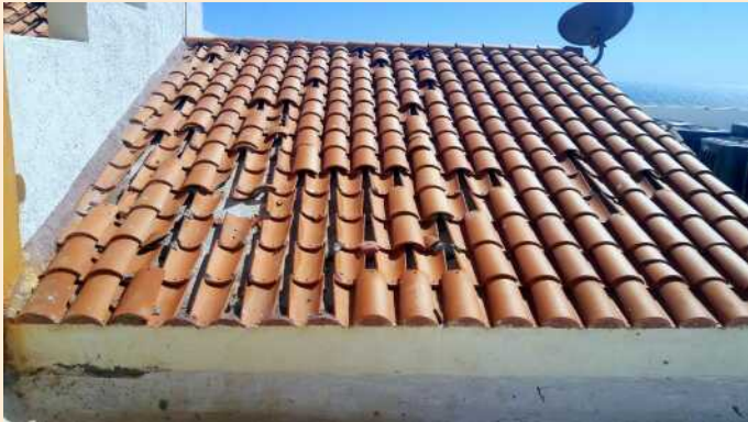
Before Tiles Replaced
