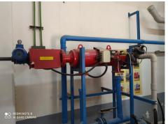
AMIAD filter is unplugged, we need to replace some components inside like the membrane and electric motor. These filter is important to remove sand and Stone particles from the Water pipes and those particles can damage all kind of valves.
