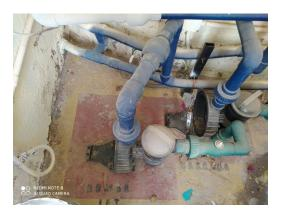
We need around 9 motors for filtering or cascades, many pumps had smart cards and these were damaged so they do not work without it.
