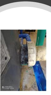
• The valve is broken and was repaired with glue only, this takes several years like this.
