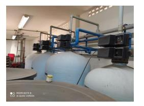
Activated carbon filters are not working, it is necessary to change the activated carbon and see the condition of the internal pipes.
