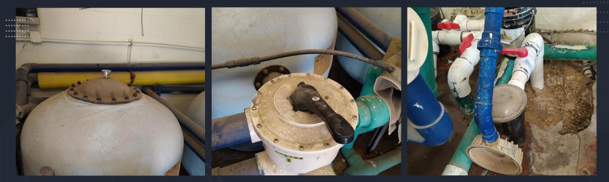
• This filter does not have sand and the valve is damaged and it is necessary to change it, the motor of this pump stopped working and that is why it was removed, currently we need 9 motors for the filter rooms, either for waterfalls or for filtering
