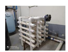
• the irrigation system when it is in use the pump is always on due to the fact that it does not have a tank that pressurizes the system and that generates more electricity expenditure, this can cause more wear and tear on the equipment.
