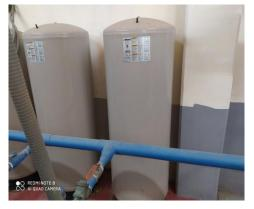
We need to replace one Hydropneumatics cylinder due the bladder is ripped off.
