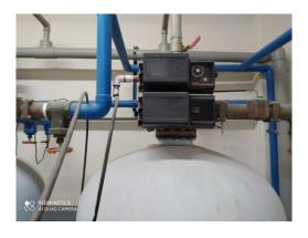
Salt Filters Is not working and the valves are stuck
