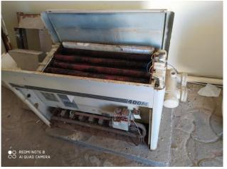
Most of the boilers are damaged and we have to replace them, some lack the pilot or are aberrated by the time of use, the heater pipes are pitted
