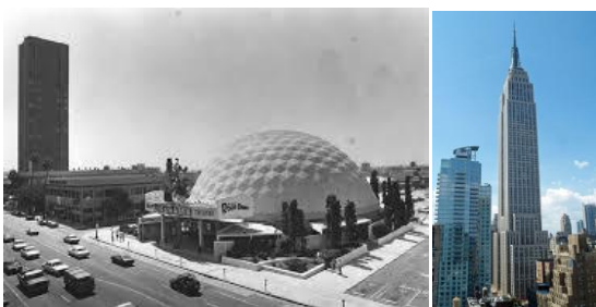
Figure 2. A geodesic dome —The Cinerama Dome Theatre on Sunset Boulevard (right in the left photograph) representing tensegrity architecture principle as compared to the high rise “vertical compression” building to its left, or The Empire State Building and its neighbor in construction in the right photograph [Internet public domain photos: www.waterandpower.org (left) and Wikipedia (right)].
