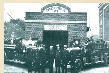
District 9 Iselin Fire Co. No. 1 1942 with 1936 LaFrance Pumper and 1923 Clinton Chemical Hose Truck
