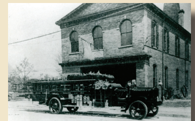
Woodbridge Fire Company Engine and Firehouse 1924
