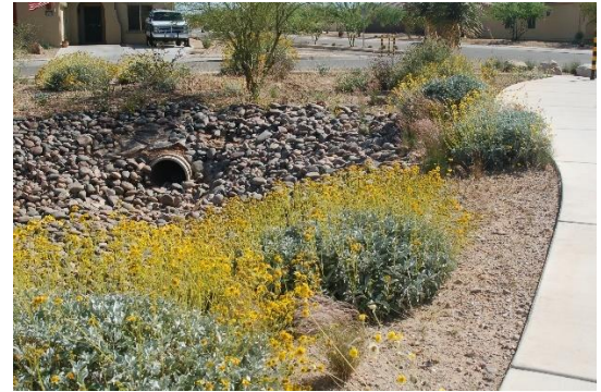
Cut Curb Water Harvesting Feature (Left) Drainage Control Incorporating Water Harvesting (Right)
