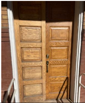
New door handle in hallway door leading to the bathrooms
