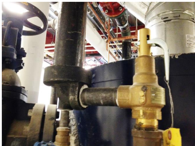
A pop safety relief valve piped into a drip pan ell.
