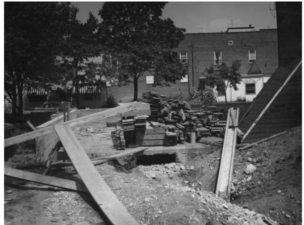
Fig. 3. Looking north across the basement and lumber towards 3 rd St. as the foundation is being finished circa September 1954.
