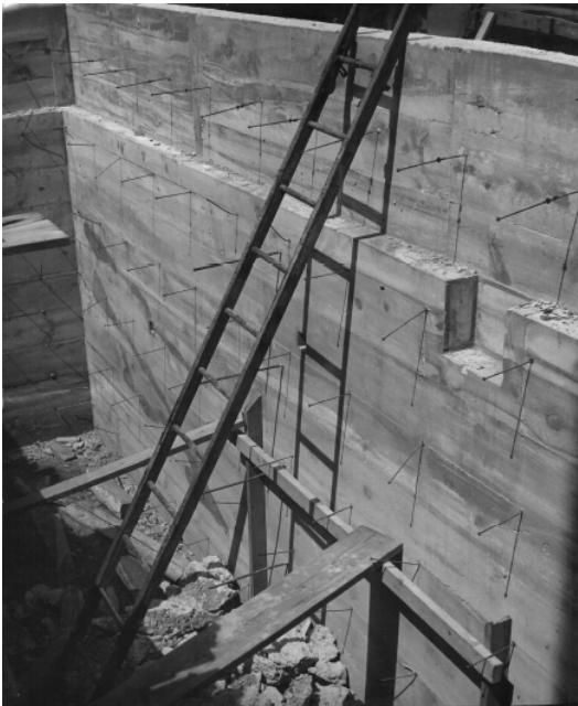
Fig. 1. Photograph of the foundation walls for the new addition taken circa September 1954.
