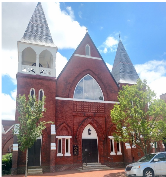
Fig. 1. Front Facade and entrance to the UMC building in Fredericksburg VA.
