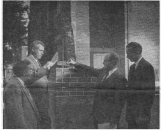
Fig. 2. Pastor H. A. Cooper is shown with two trustees and the District Superintendent at the "official" ceremony just prior to starting laying bricks on the nearly completed foundation.
