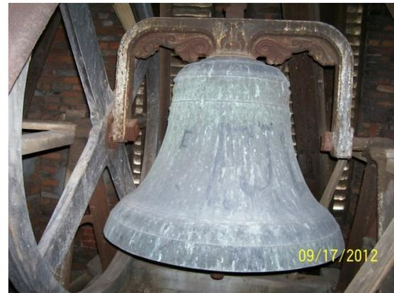
**Fig. 4. Photograph of the bronze bell in the steeple of FFUMC.**
