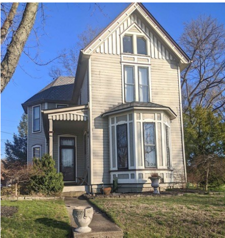
Fig. 2. The Former 19 th Century Methodist Parsonage (Photo from March 2023)
