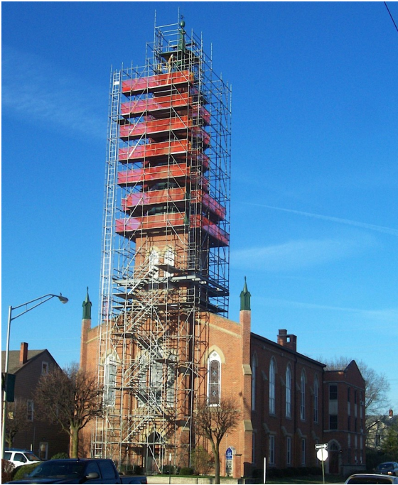
Fig. 9. Scaffolding on Steeple in December 2011.
