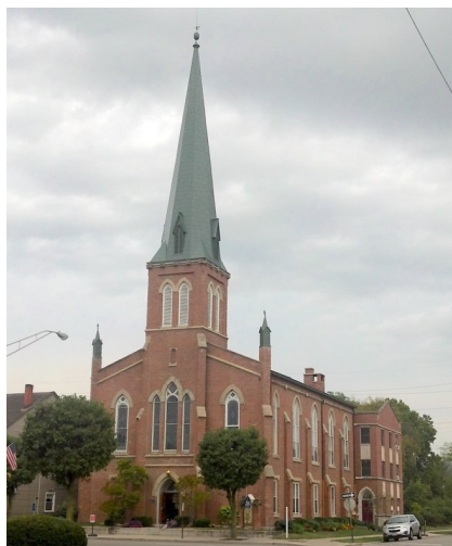
Fig. 8 View of FFUMC in September 2012.
