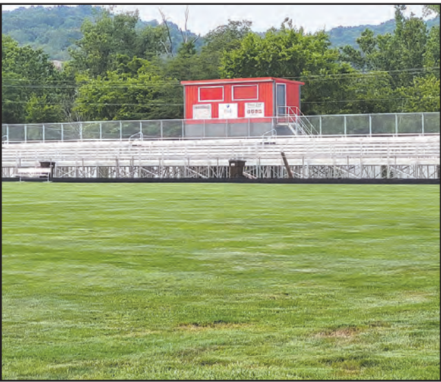
Installation of new visitor-side bleachers at Loudonville High School's Redbird Stadium was recently completed. The previous bleachers were deemed deteriorated and unsafe and were replaced by the Board of Education this summer, with part of the cost covered by a $60,000 donation from American Legion Post 257.
