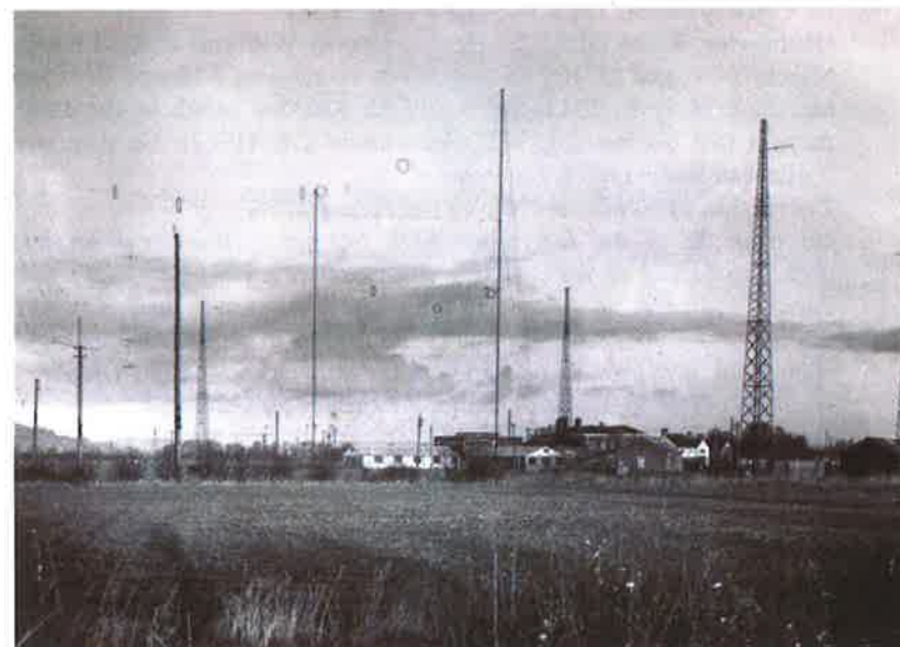
Portishead Radio Masts. Courtesy of British Telecom
