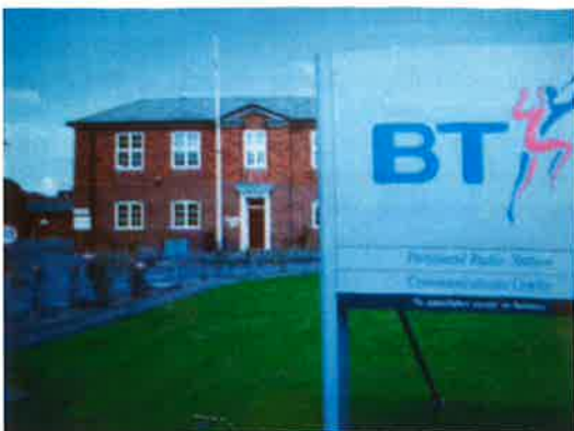
Portishead Radio main building.
