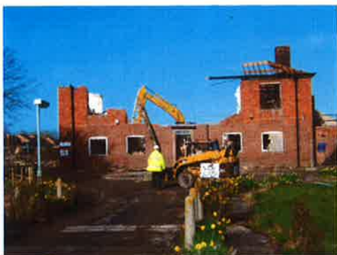
Portishead Radio main building during demolition.
