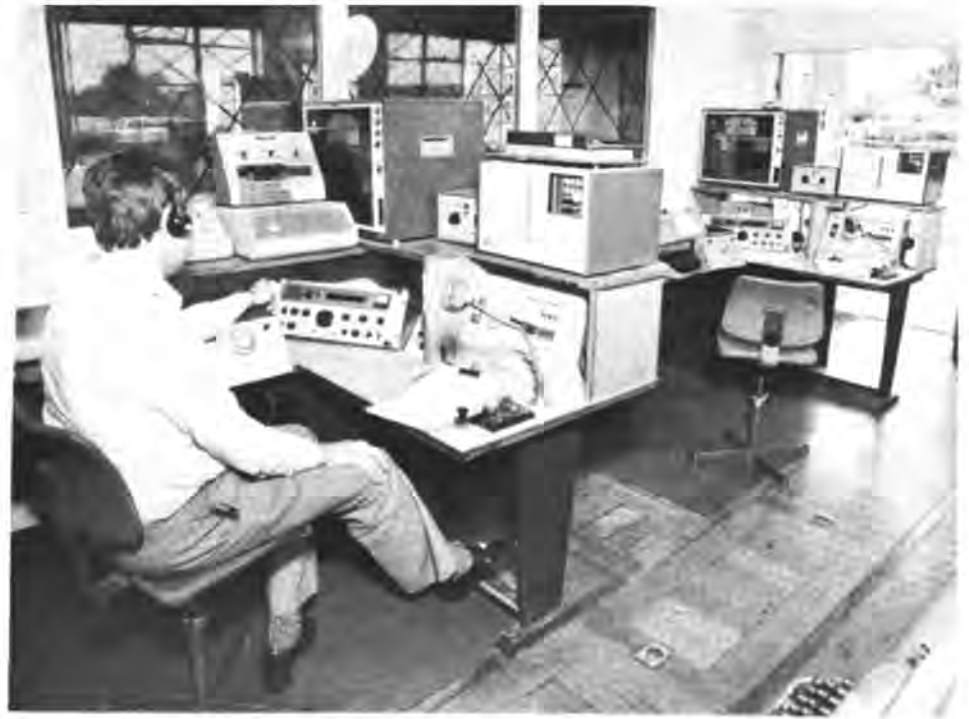
PART OF THE RADIO TELEX ROOM - Chris Hammond Studios Picture.
