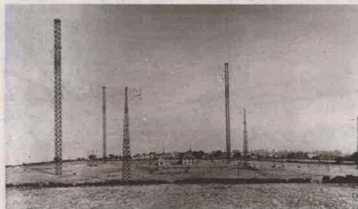
The Portishead transmitter site, c. 1933
