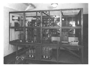
The Main receiver was a Marconi Type 12A direction finding receiver used for the main 600-metre band.
