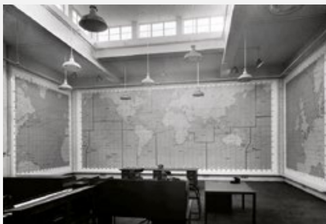
CONTROL ROOM SHOWING STEEL WALL MAPS, 1948.
