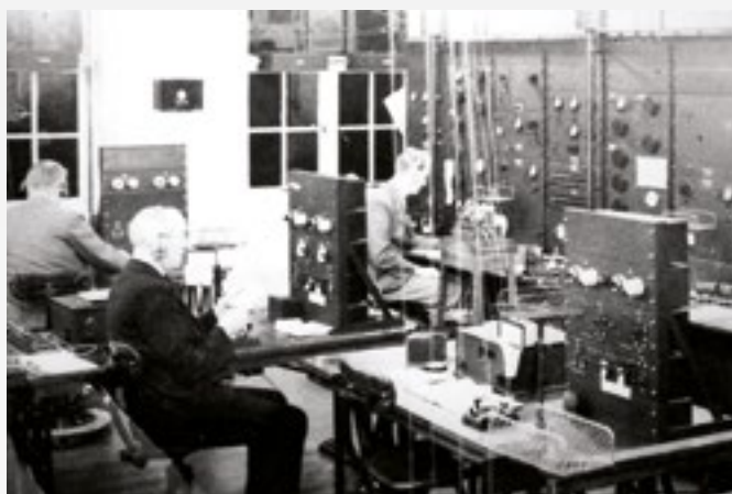
A SECTION OF THE HIGHBRIDGE OPERATING ROOM, 1938.
