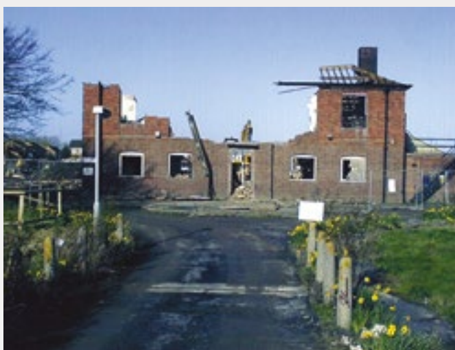
THE DEMOLITION OF THE STATION ENTRANCE BUILDING, 2007.
