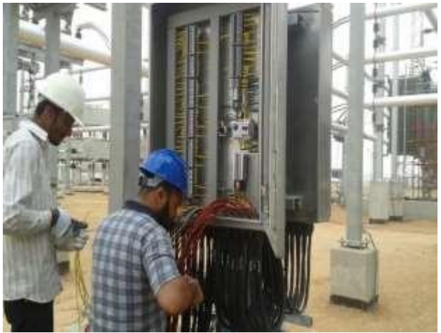
Outdoor yard termination work
