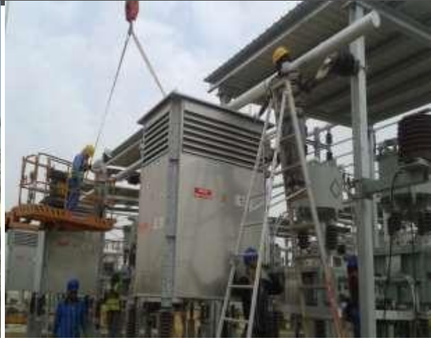
Aluminum Busbar Installation at filter
